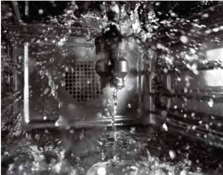
Automatic cleaning system
